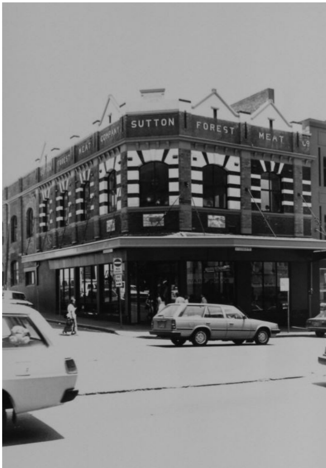
Image shot in 2000, depicting the heritage facade & its ceramic tile patterns (1231). Malaya Restaurant. City of Sydney Archives
